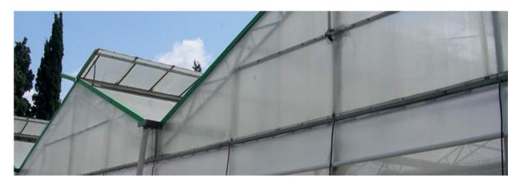
Specially manufactured with a clear tint appearance, provides excellent thermal insulation, highly flexible, yet virtually unbreakable, rigid sheet structure provides extra strength under wind and snow loads.
