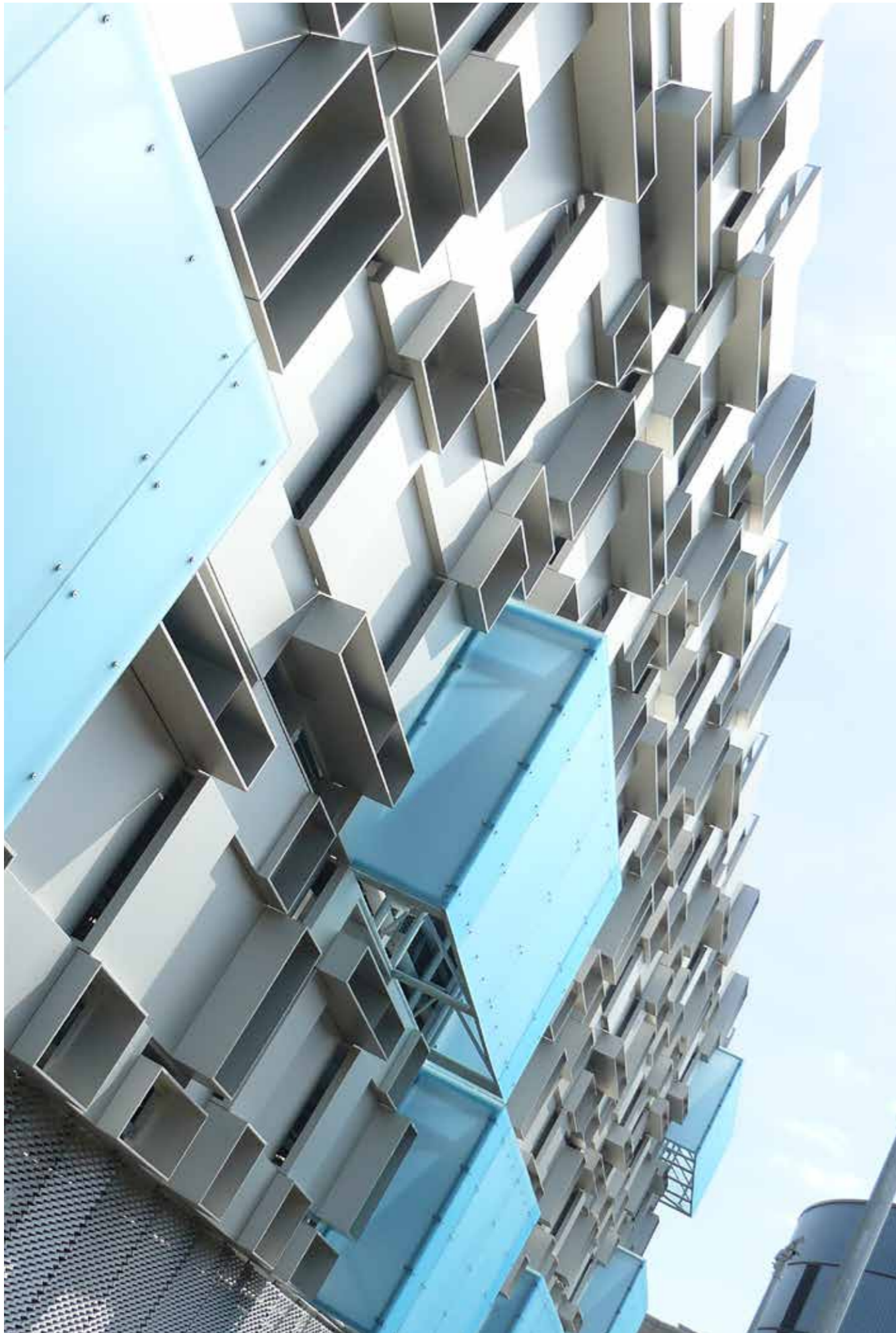
Car park facade using PERSPEX® Frost Arctic Blue S2 7T77 | ©Photograph: Image Technique
