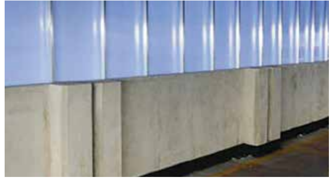
CAR PARKING STRUCTURES
